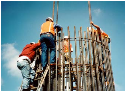
Reinforced Concrete Inspection
