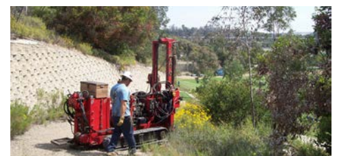
Limited Access Drilling
