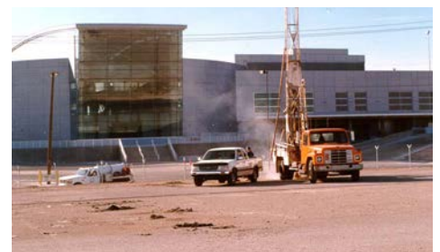
Las Vegas McCarran International Airport
