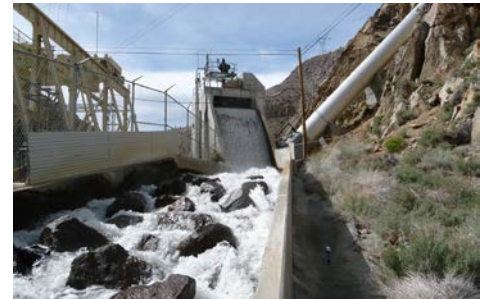
Upper Gorge Hydroelectric Power Plant
