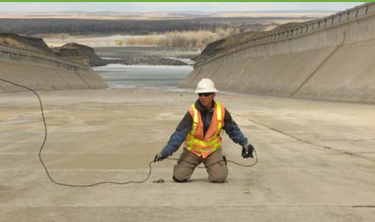
Fort Peck Dam Spillway
