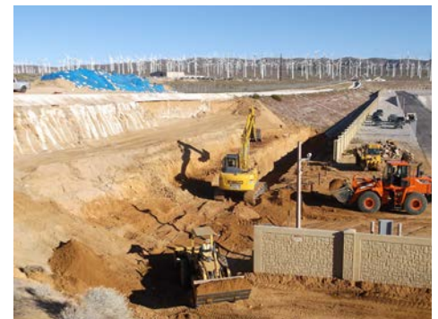
Windhub Substation Slope Repair
