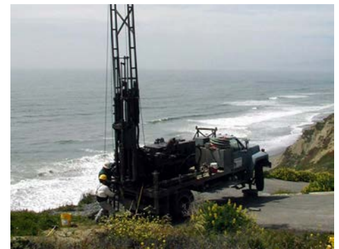
Avalon Canyon Slope Repair
