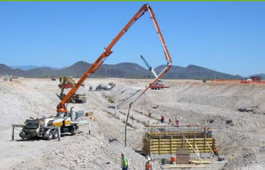
Lake Pleasant Wastewater Treatment Plant
