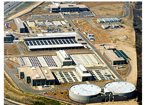
North City Water Reclamation Plant
