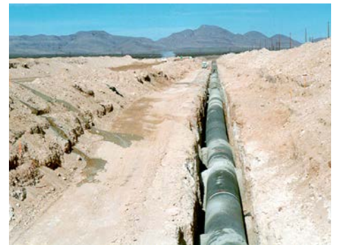
East Valley Lateral Pipeline
