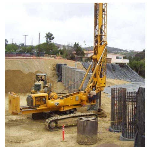
Shear Pin Installation
