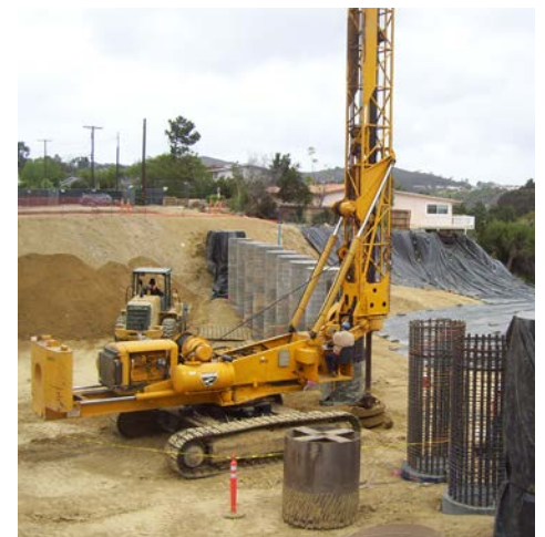
Shear Pin Installation
