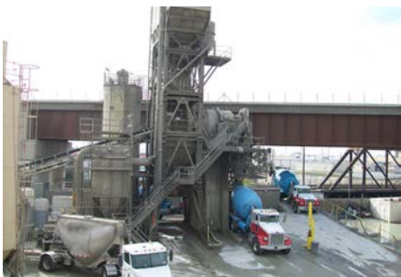
Concrete Batch Plant Inspection
