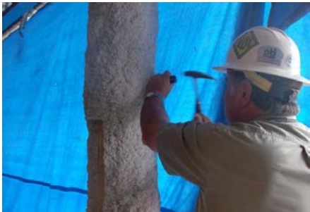
Fire Proofing Inspection
