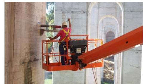
Forensic Core Drilling
