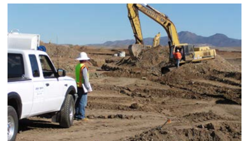
Utility Trench Backfill
